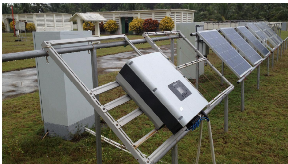
Outdoor testing of Huawei inverters is conducted at a location which is frequently hit by typhoons and sees temperatures exceed 40^{\circ}\text{C} during the summer months.
