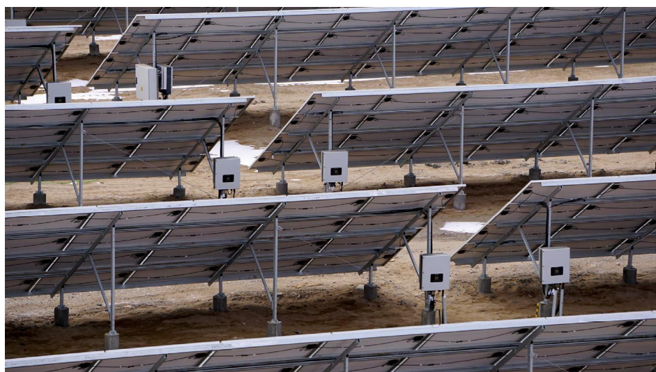
Huawei inverters at a 590 MW PV project in Qinghai Province, northwestern China.
