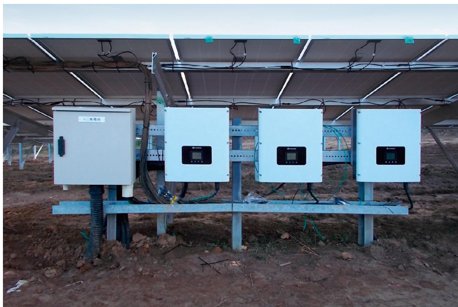
Huawei inverters installed at a ground mounted PV project in Japan.
